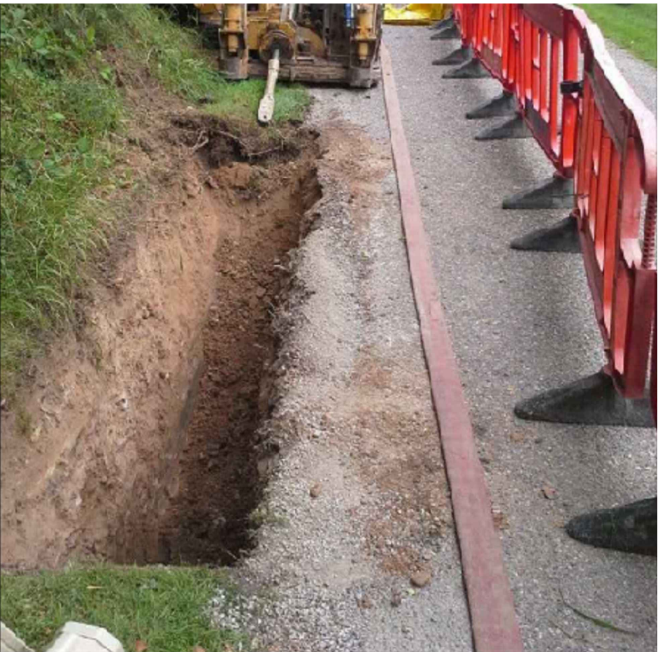
TYPICAL DRILLING RIG & LAUNCH PIT
